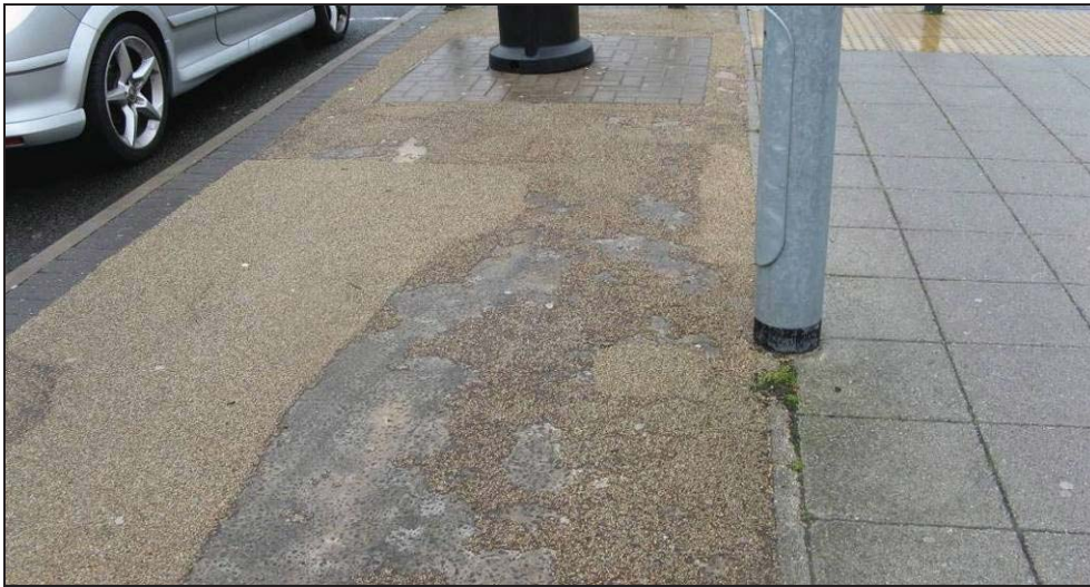
Figure B.7 – Resin bound gravel in poor condition at Norton Canes MSA
