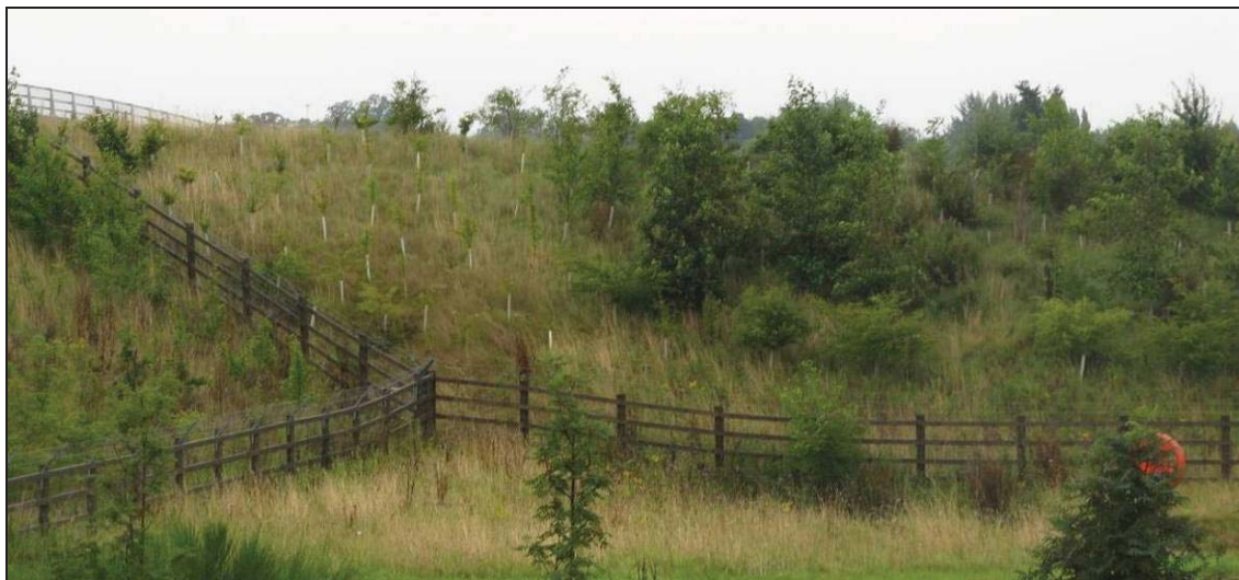
Figure B.3 – Area of poor vegetation establishment on embankment near Wishaw
